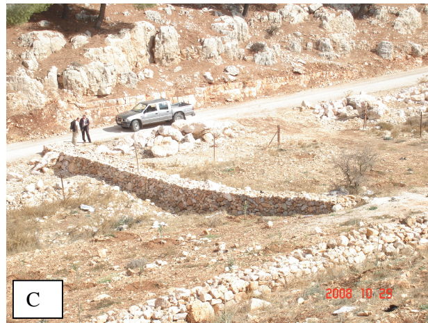
Appendix F. Photo 18: Soil conservation structure (dike) across the wadi.
